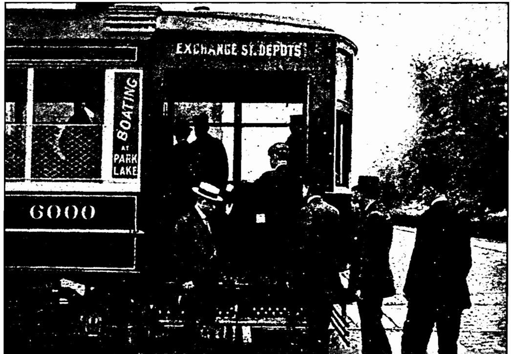
*One important innovation in use by 1911 was the "nearside car" which permitted passengers to enter and exit only by the conductor. This allowed the conductor to stay in one spot and still collect fares.*
